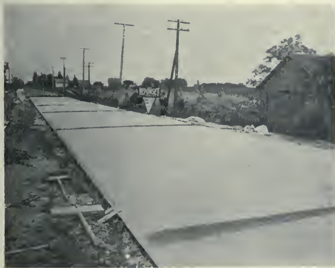
Fig. 1.—Expansion joints are placed every 35 ft.
